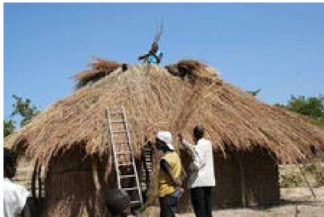
Villagers helping to build Florinda's new home
